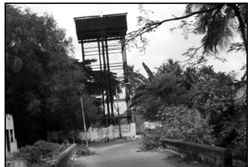
Old overhead water tank
