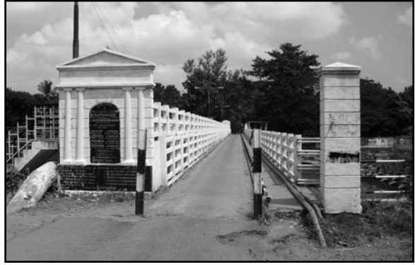
A view of bridge on Arasalaru on the periphery of Agalankan
