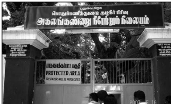
Water pumping station in Agalankan
