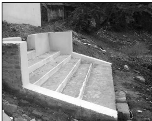
Construction of steps nearing completion
