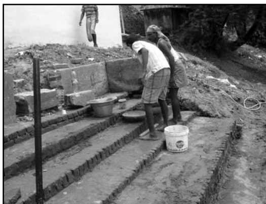
Steps under construction in the village pond
