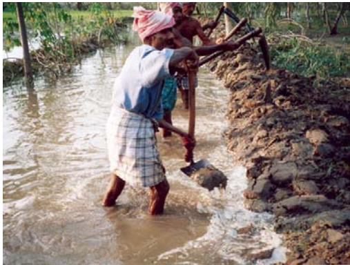
Desilting the irrigation canal
