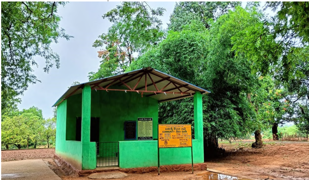
▲ Community Seed Bank at Ramaguda
