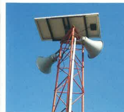
GSM-based public address system
