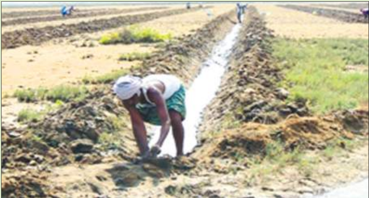
Digging of canals for tidal water flushing
