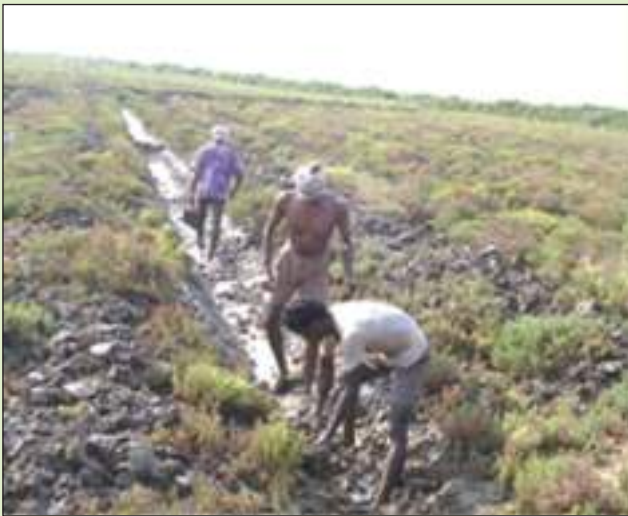
Desilting of canals for facilitating tidal water flow
