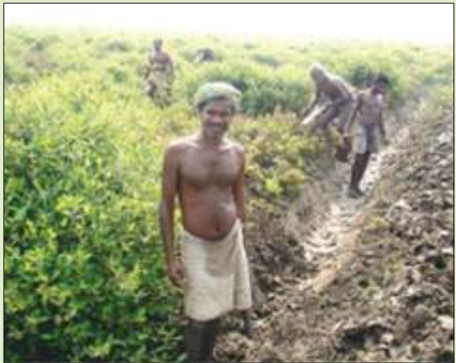
Desilting of canals for facilitating tidal water flow
