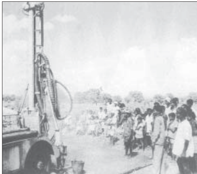
Photo 8.1: One of the Early Drilling Rigs
