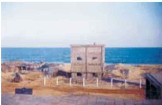
Photo 8.4: Narippaiyur Intake Point
