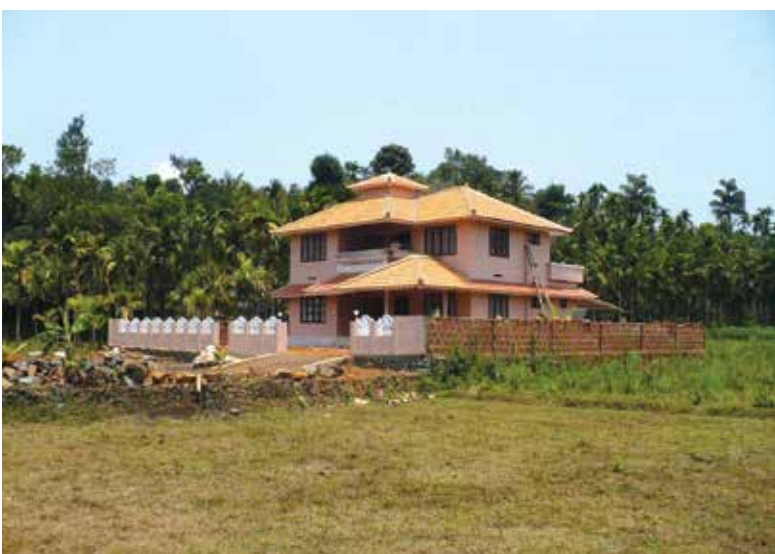
Figure 7. Conversion of paddy field for housing purpose (Photo by Prajeesh Parameswaran)
