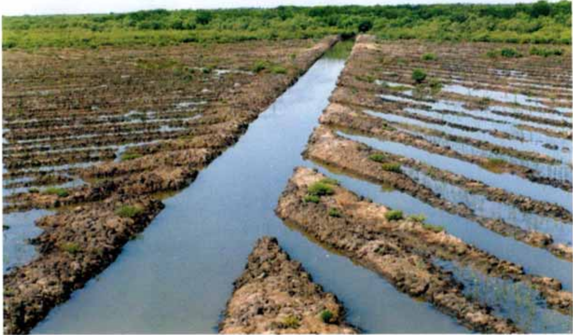
Fish bone type canal as dug in one of the restoration sites in Pichavaram mangrove wetland of Tamil Nadu
