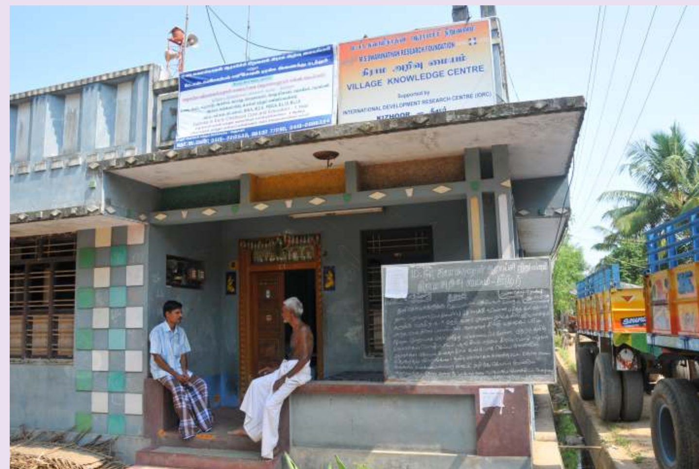
Mr. Jayakrishnan and his father at the entrance to the VKC located in the front section of their home
