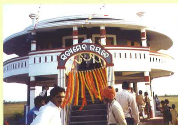
Multi-purpose cyclone shelter set up in Gyaspur, Orissa.
