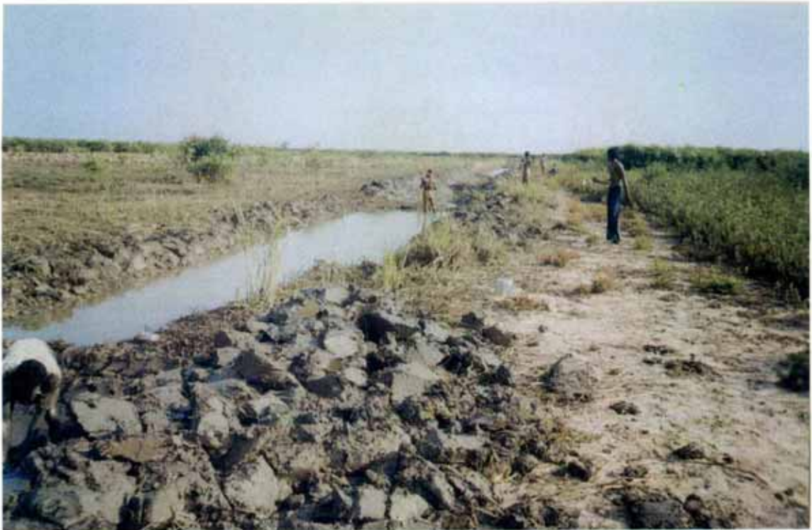
Figure 22. Digging of canal for restoration
